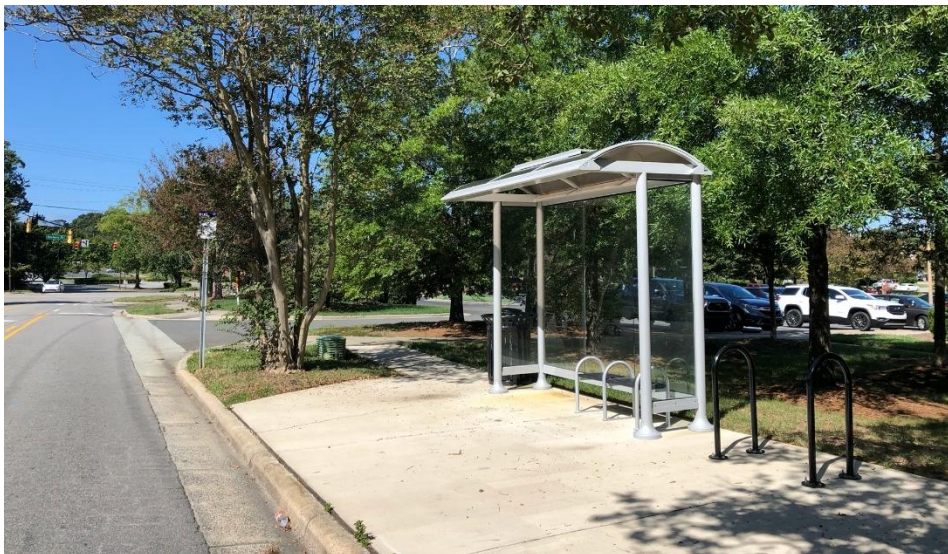
Example of stop near driveway.
