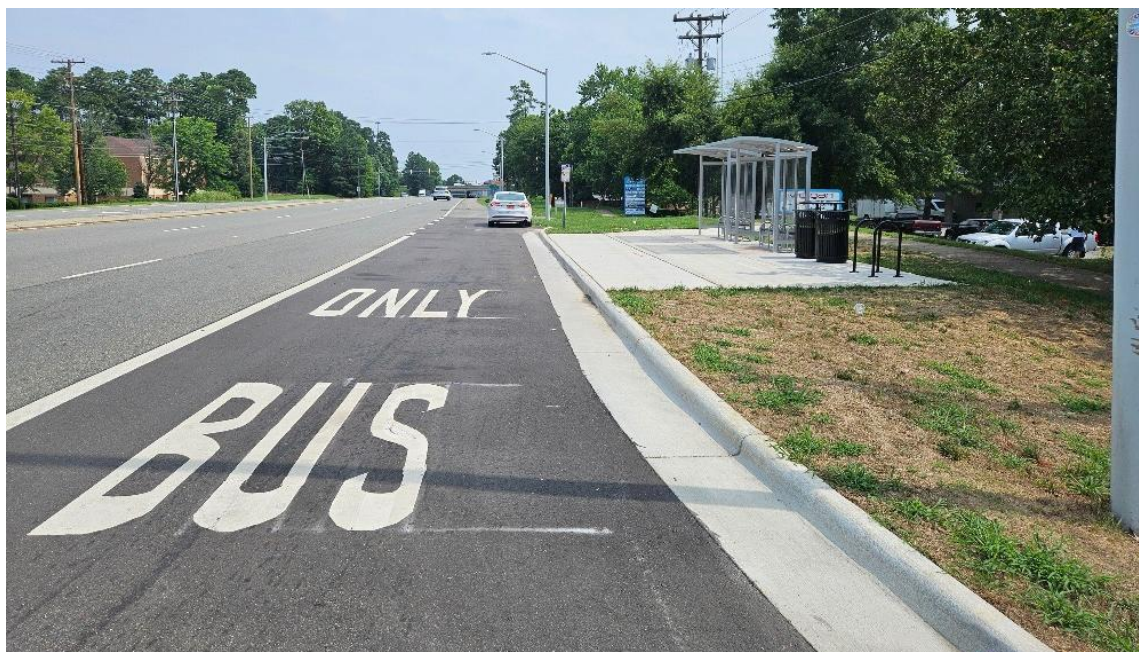
Example of bus bay.
